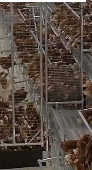
zones with moon lighting atop and under-lights below, this system provides a nurturing environment for the birds, enhancing their well-being and productivity. The light dimmers are a CBM 48v system with 12 watt lights that contain a 8 watt white and 4 watt red that can be custom blended for infinite color temperature. This system is integrated into a custom United Agri Systems control panel to allow the lights to run on a schedule to optimize the health and productivity of the birds.
